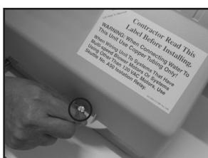
3. Disengage the humidifier cover from the mounting frame by rotating the thumb screw at the bottom counterclockwise (→).
