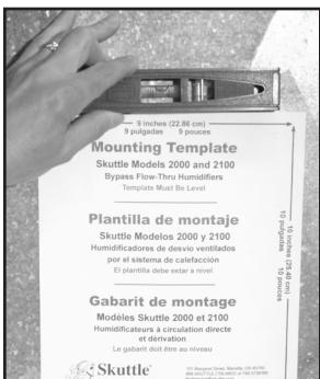
1. Locate the 2000 or 2001 mounting template in the humidifier carton. Tape the template lengthwise onto the furnace plenum, **making sure it is level**.
