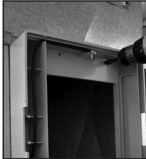
7. Place the mounting frame into the plenum opening so that the frame hooks over the bottom of the opening. Screw the frame to the plenum.
