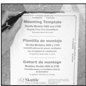
2. Trace around the template.\* Remove the template. Accurately cut the plenum opening.
