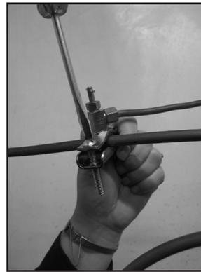
**12.** Tap into the water supply line using the saddle valve provided. Follow the directions on the saddle valve bag.
