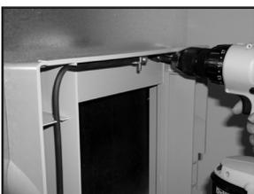
6. Place the mounting frame into the plenum opening so that the frame hooks over the bottom of the opening. Screw the frame to the plenum.
