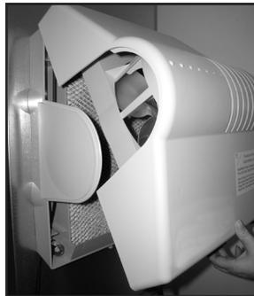
9. Reattach the cover assembly by hooking it at the top of the mounting frame. Secure the cover by turning the thumb screw at the bottom clockwise (↻).
