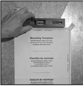
1. Locate the 2002 mounting template in the humidifier carton. Tape the template lengthwise onto the furnace plenum, **making sure it is level.**
